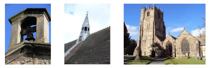
Fig. 2. A stone turret above a gable end, a flèche midway along a roof apex and a massive masonry tower
