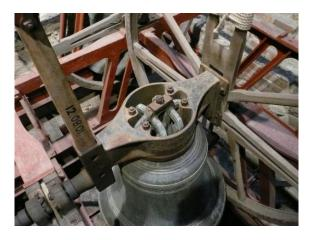
Fig. 8. Canons, iron straps and wooden headstock and a steel canon-retaining headstock
